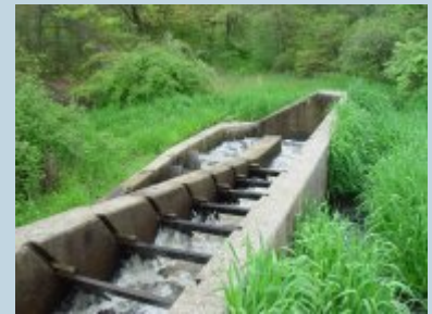
Bradford Fish Ladder, a denil-type fish passage structure on the Pawcatuck River in Bradford, R.I.
