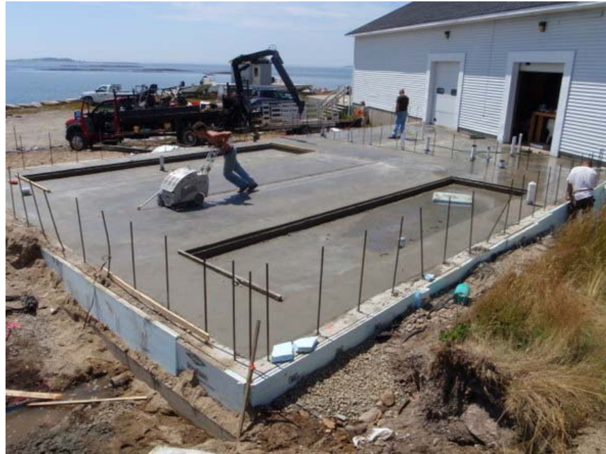
DEI's Marine Education Center under construction (July 21, 2010)
