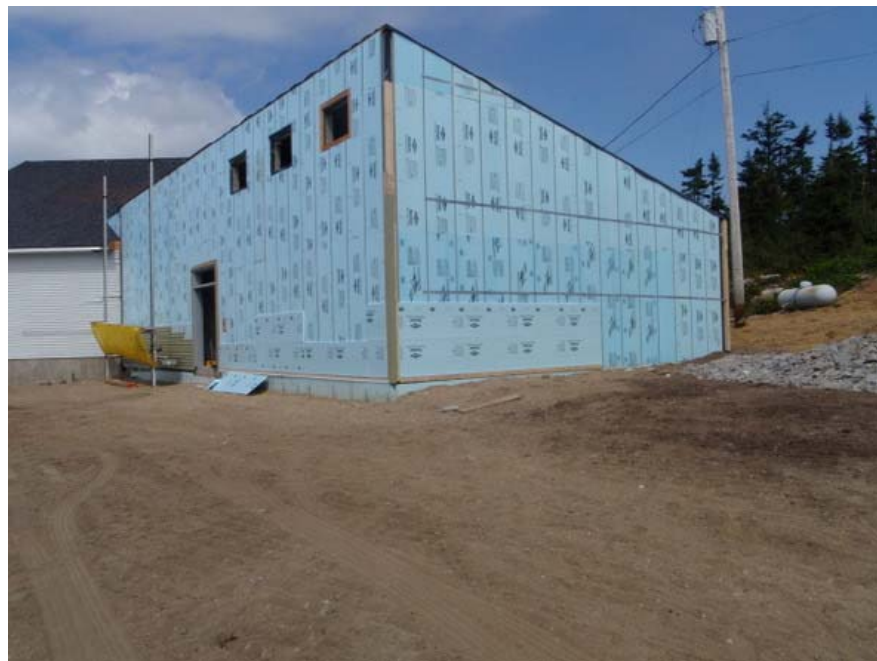
DEI's Marine Education Center under construction (August 20, 2011)
